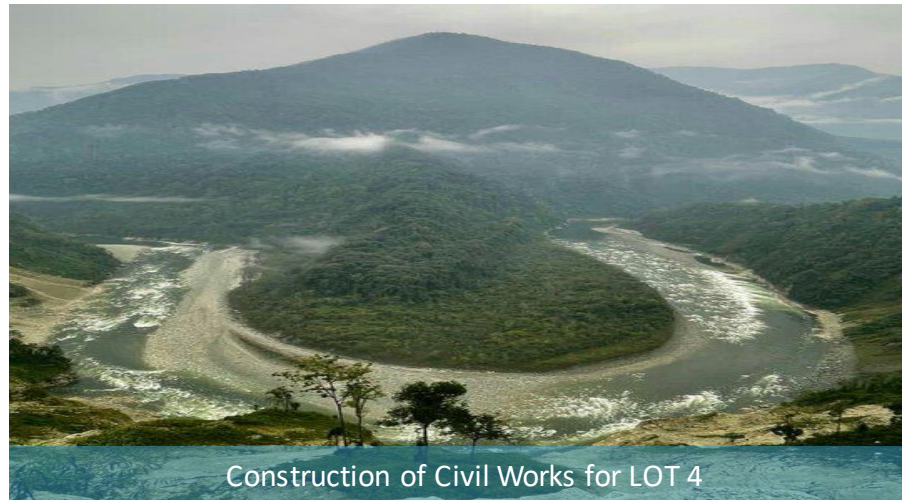
JV - DIBANG POWER PROJECT (ARUNACHAL PRADESH)
