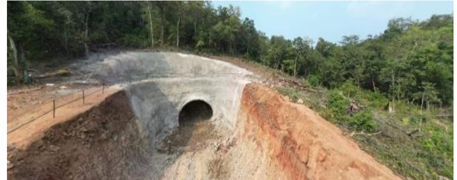
4 Tunnels on new railway line ( 7.49KM)
