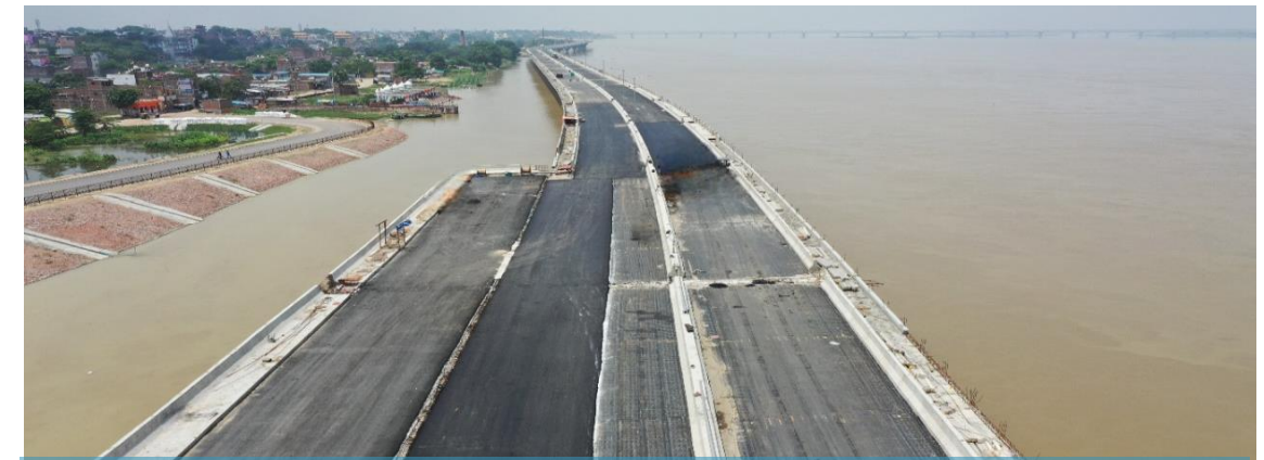
Four lane elevated road (4KM)
